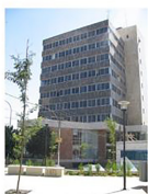
The insurance building, an example of Amman's International Style/Curtain Wall Public Buildings typology
