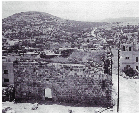
Exterior and interior views of the Zaidani Mosque of Tibneh in northern Jordan. The roof of the mosque has been severely damaged after the 1927 earthquake. The mosque, stands deserted, still waiting funding for its rehabilitation.
