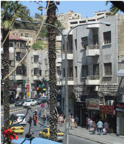
Figure 5. Exterior view of the former Islamic Bank on Faisal Street showing the building in its original simple Ammani style before the removal of the cantilevered verandas and the addition of the neo-classical motifs.
