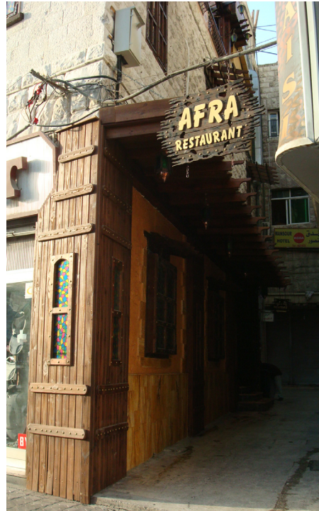
Figure 4. Exterior view of the entrance to Afra restaurant from the side alley on Faisal Street in Downtown Amman showing the excessive usage of wood cladding, brass, and historic lanterns.
