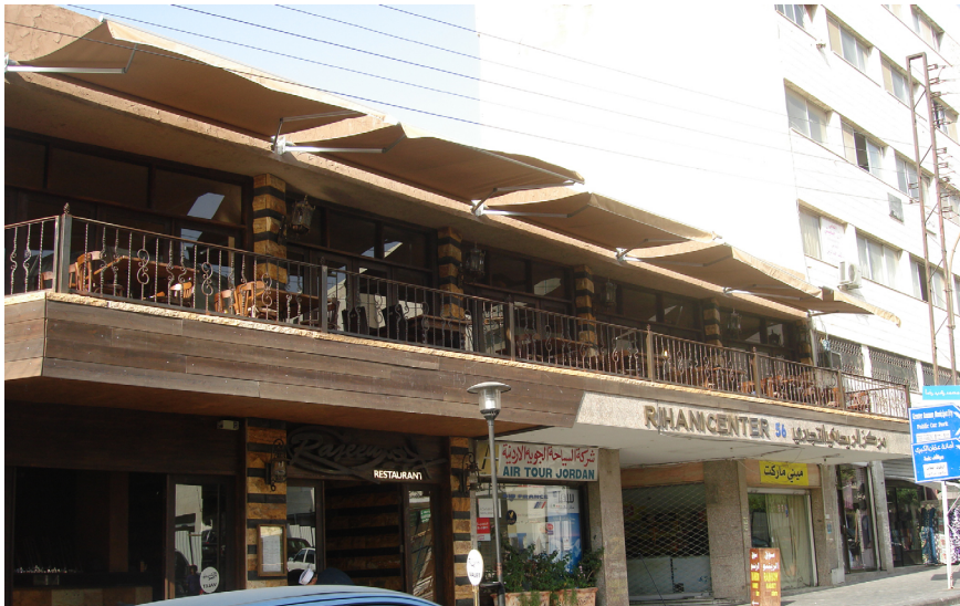
Figure 1. Exterior view of Raje'en restaurant on Rainbow Street showing excessive usage of wood and stone cladding over original gray marble facades from the 1960s.
